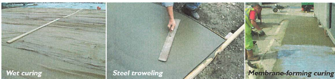
Prevention measures for concrete crazing
